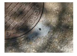
7. Insert the 12mm wide x 80mm long Fundilock union plug into the hole and press it so that it is incarcerated until it reaches a perfect leveling with the cover. Then, wait for it to set.
