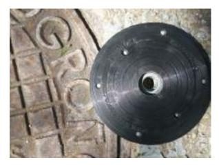
8. Place the neoprene washer and just above the polypropylene Fundilock washer, both aligned with the already set union plug. Take into account that the union plug is composed of a threaded rod welded to a socket that allows an insertion up to 25mm.
