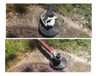
11. To tighten we can use both a wrench or a torque wrench. It is recommended a tightening torque of 44Nm.
