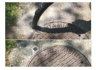
5. We vacuum the dust produced during drilling to clean the hole.
