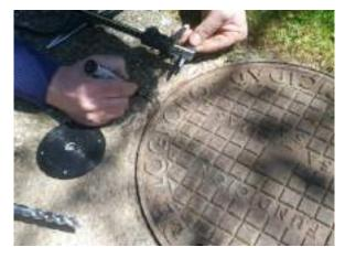
3. We look for the flattest area next to the lid and mark where we will make the installation holes, in such a way that we save the frame and block the maximum possible surface of the manhole cover. In this case we make the mark at 50mm from the point to be protected.
