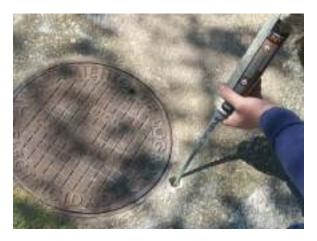
6. Fill the hole with bonding material (chemical block, chemical blister or cement for anchors like sikadur).
