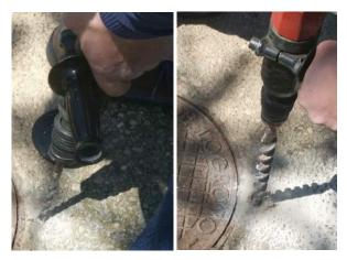
4. Drill vertically, first with a drill bit of 12mm to 100mm deep. Subsequently, we increase the hole with a 25mm drill bit for concrete.
